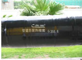
The surface should smooth, no gauffer, no gas bubble after the tubular sleeve is shrunked and the tubular sleeve should adhibited to the weld and the slope of two ends of primer anti-corrosion layer firmly.
