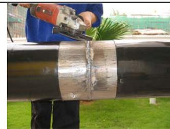
3 Clear up all the bur, splash, rust, oil, dirt and any other sundries with an electromotion tool (steel wire brush)
