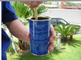
7 Mix solvent-free two component epoxy primer (pour B to A) and mix round the mixture for 3-5 minutes
