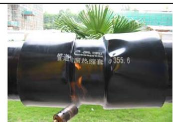
11 Heat the sleeve from the middle part round the sleeve equably to make the middle part shrink firstly and then heat another end of the sleeve from a round direction to make sure eliminate all air bubble and the heat-shrinkable sleeve is shrunk onto the steel pipe firmly
