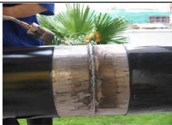
2 Preheat the weld to 30-40°C to eliminate the vapor (dew or frost) around it with a blowtorch
