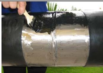
8 Paint the primer on the pipe surface equably using a special dope brush, thickness  $\geq 150\mu\text{m}$  (the mixed lacquer should used up in 1 hour)
