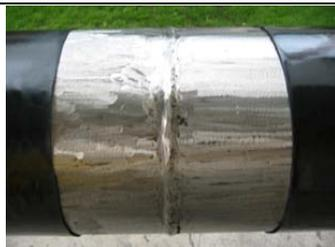
4 The standard of de-rust should up to Strate (de-rust using electromotion tool); GB8923Sa2.5 (de-rust using sandblast). The gradient of processing for the end of anti-corrosion layer should no more than 30 degree
