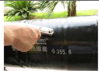
15 Press the unevenly surface of the tubular sleeve with an idler wheel
