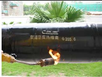
14 When the two ends of the tubular sleeve shrink drastically, heat the sleeve from round direction again using a small fire to make sure the adhesive melt and firmly adhibited.
