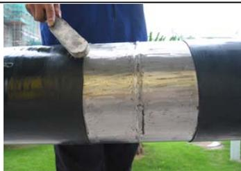
5 Granulate the two sides of the weld and the lap joint of the anti-corrosion layer and then eliminate the ash after finishing eliminating rust (no more than 2h until welding)
