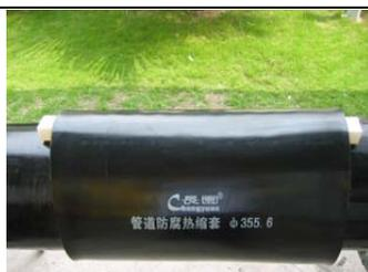
10 Set a certain height of chock inner the tubular sleeve to make sure the sleeve has some tensile force
