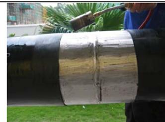
6 Preheat the weld and the lap joint of anti-corrosion layer to 55-65°C
