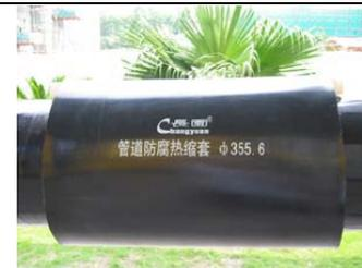
9 Install the sleeve to the middle of weld quickly and make sure the same width of the two lap joints on to the anti-corrosion layer, and the width should equal to or more than 100mm. Press the two lap joints using an idler wheel to cling firmly
